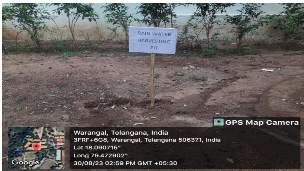
Fig: Rain Water harvesting pits
