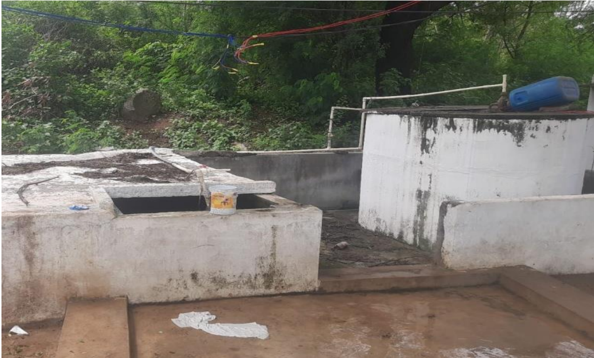
RO waste water storage sump
